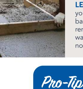
your form, level (screed) the concrete in a smooth back-and-forth, sawing motion, making sure to remove excess concrete and fill any voids. If a water sheen appears on the surface, this is normal and can be ignored.
