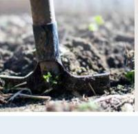
**EXCAVATE** For a pad to sit 2" above ground level, you'll want to excavate roughly 6". Make sure to remove enough soil outside of your marks to accommodate formwork, 4" should do the trick.
